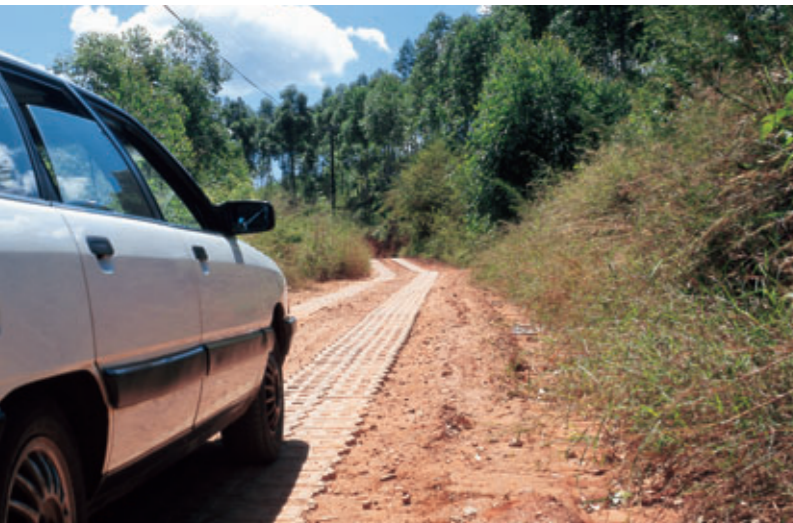
Armorflex as strip road in forest area
