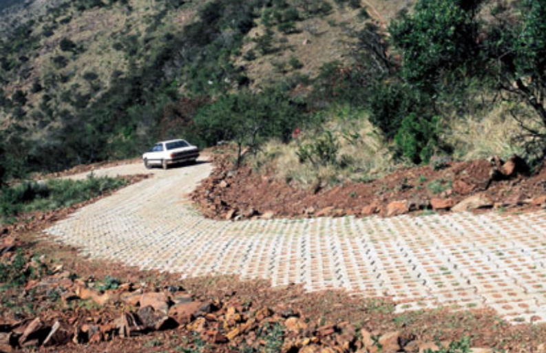
Full width Armorflex surfacing on very steep road
