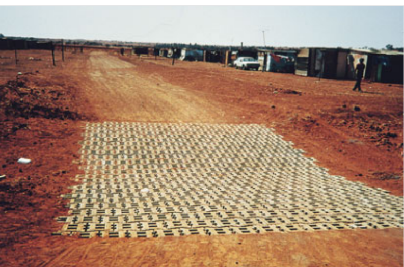
Armorflex lined stormwater crossing of gravel and surfaced roads
